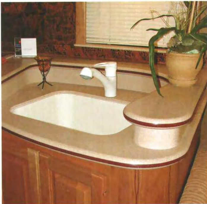
Thermoforming proved to be useful in the edge treatment seen here.
